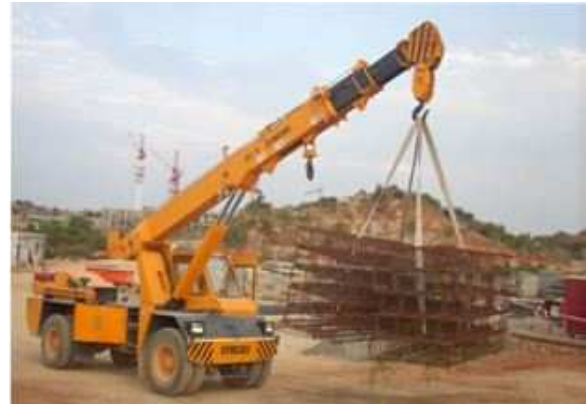
Figure - 5: Steel Frames Lifting
