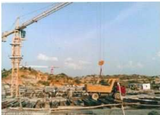
Figure - 3: RCC Columns Loading in the Trailer
