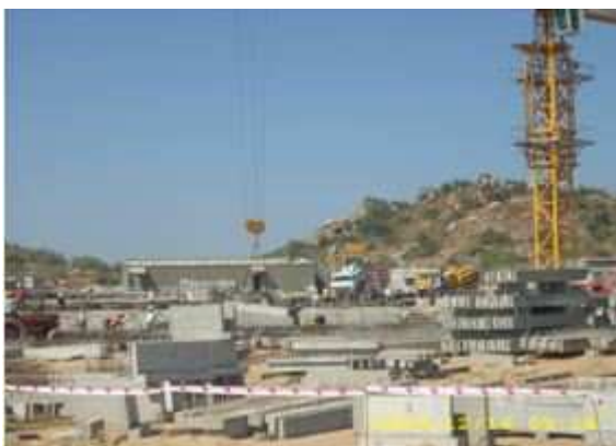
Figure - 4: RCC beams lifting
