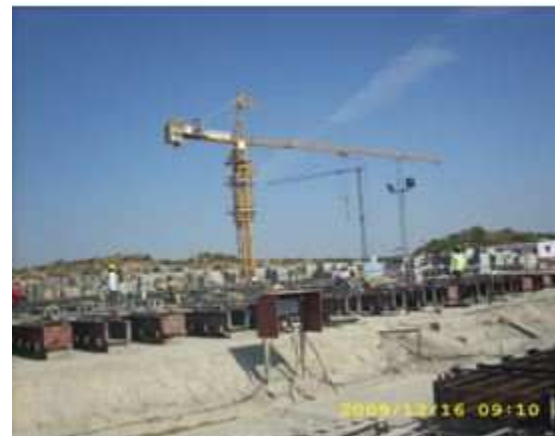
Figure - 6: RCC Columns lifting
